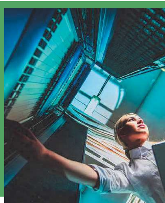
Picture supplied by Schneider Electric
